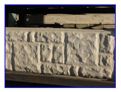
High quality pre-cast gravel board made using superplasticiser
