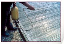
moisture in the concrete in the first 72 hours improving the concrete's strength.
