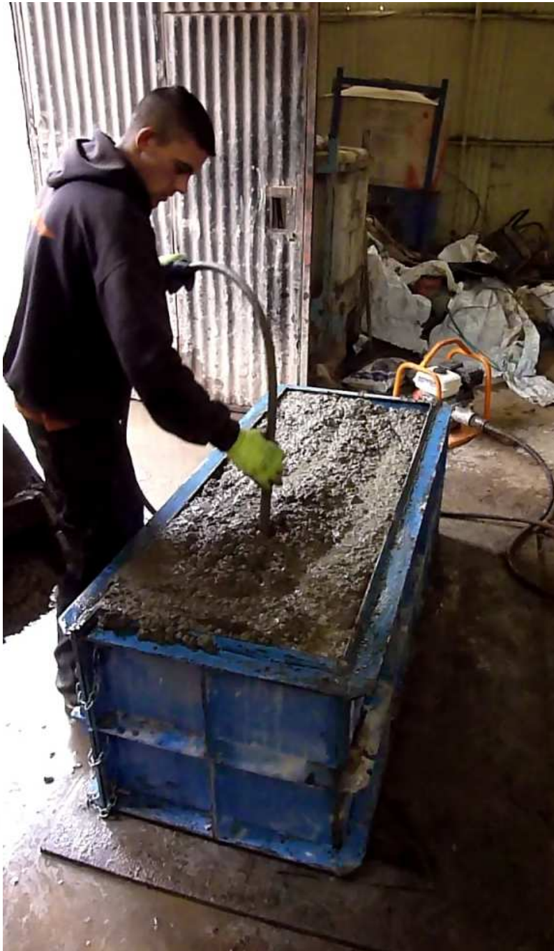
Compacting the top layer in an Armcon Surefit block mould
